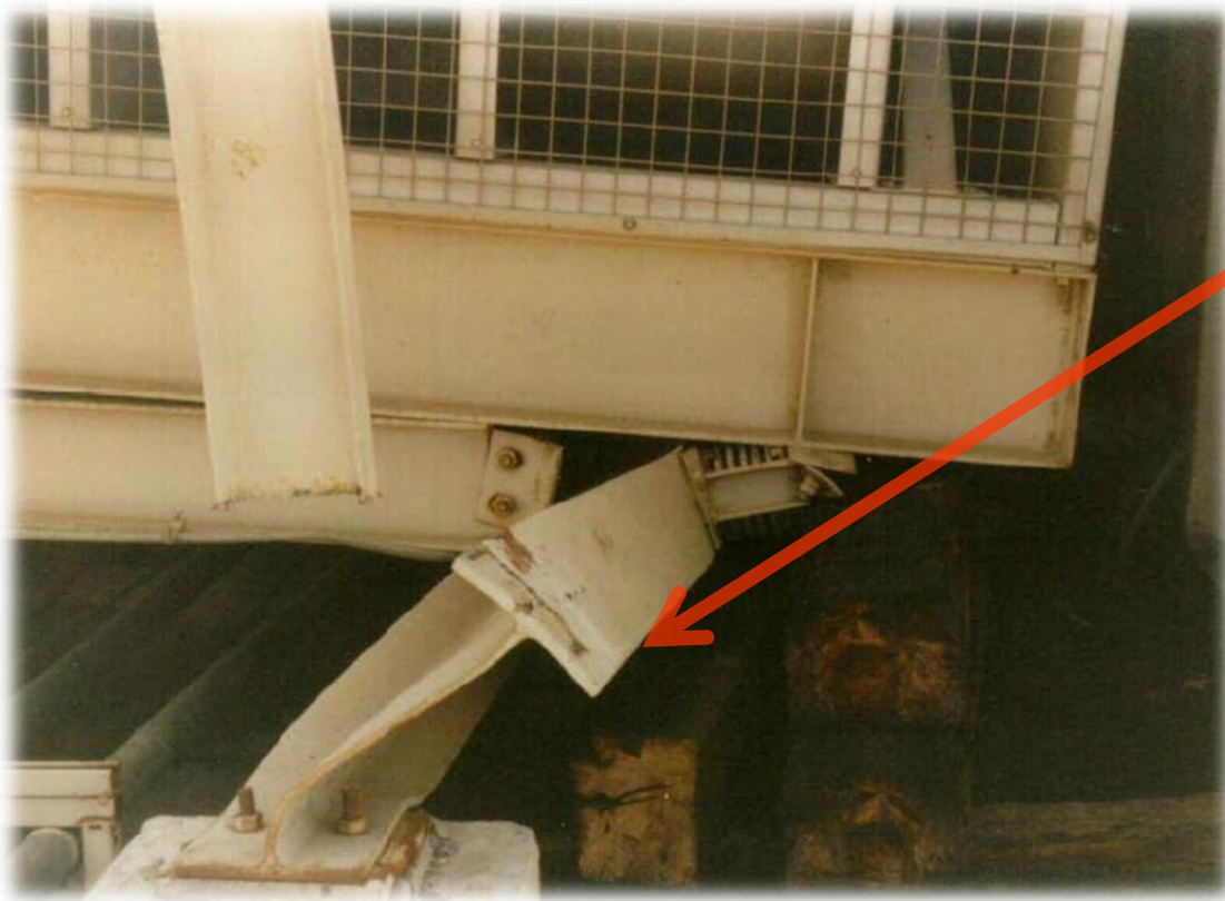
Example of resiliently (vibration isolated) mounted equipment failure (Photo courtesy of Mason Industries)
