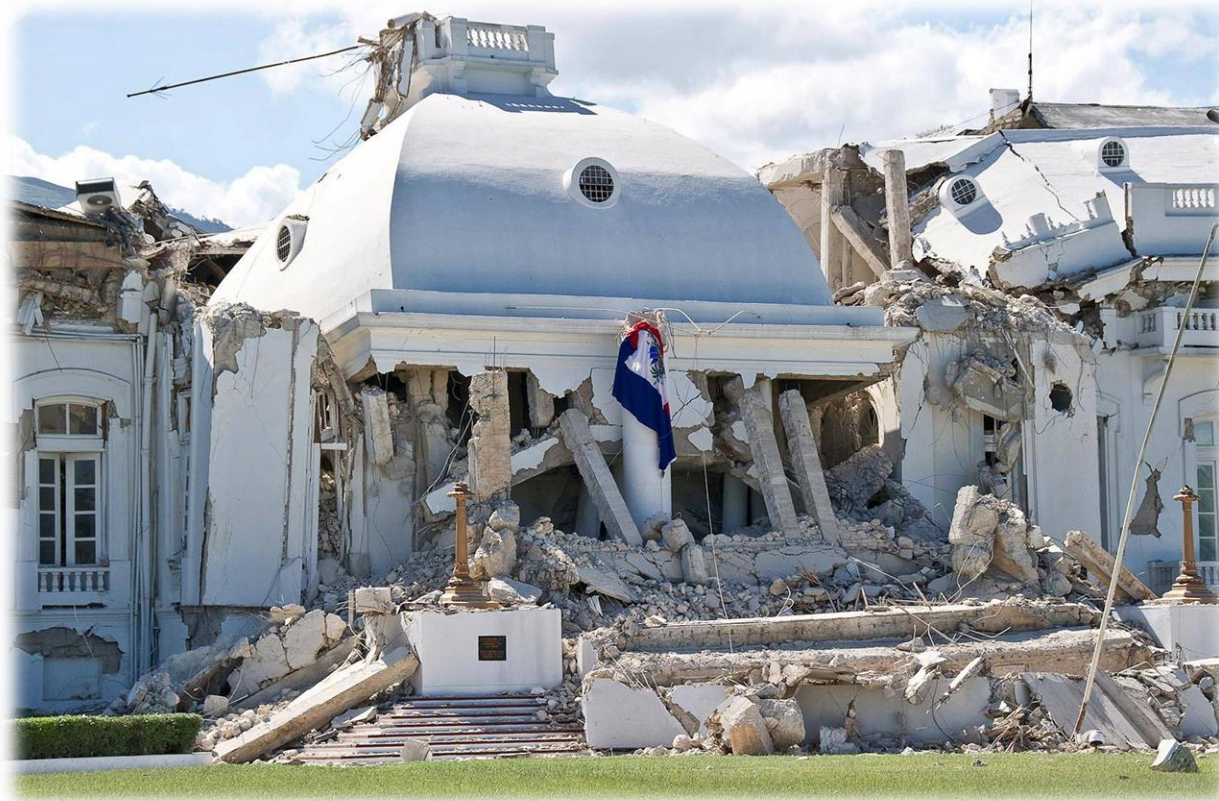
Haiti Government Palace Suffered major damage that was beyond repair
